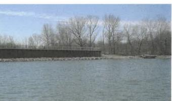
This major \$2.9 million project involved removal of 800 linft of failed steel sheet pile retaining wall and existing tieback system and replace with a new steel sheet pile retaining wall, soldier pile and deadman tie-back systems, Armor stone toe-protection, perimeter fabricated wooden fencing storm sewer and drainage improvements and general site restoration.
