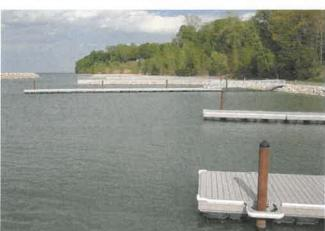
Construction of new recreational marina for the Village of North Perry, Ohio. Manufacture and placement of 39,900 tons of stone to construct two (2) aggregate breakwaters and one (1) aggregate groin. Construction of steel bin wall piers with Cast In Place concrete decks, new floating docks, Cast-In-Place concrete sidewalks, asphalt pavement parking lot, storm sewers, lighting and landscaping.
