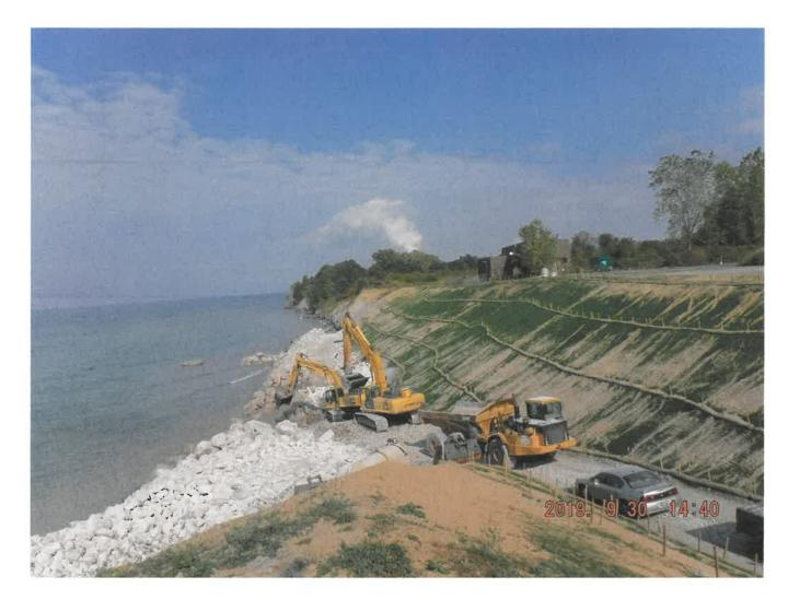
This major \$3.4 million project involved Excavation and disposal of approximately 11,125 cuyds embankment and Quarrying, Trucking and Placing approximately 21,650 tons of limestone Armor Stone, Underlayer Stone and Bedding Stone to reshape, stabilize and protect the deteriorated embankment adjacent to one of Lake County's water intake structures. Additional work included new cast in place concrete manhole and construction of a new access road.
